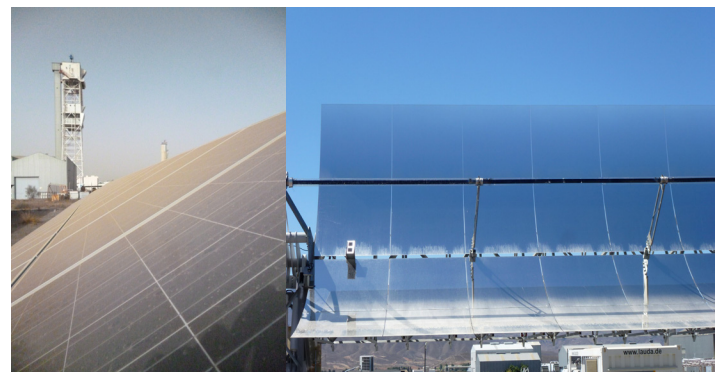
Figure 16. Soiled PV panel (left) and CSP trough (right)
