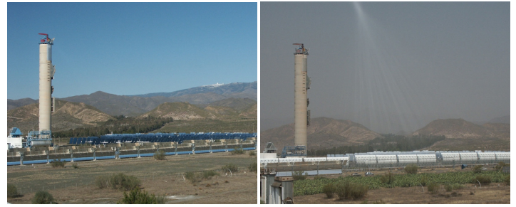
Figure 18. CSP tower plant CESA1 at the Plataforma Solar de Almería on a clear (left) and hazy (right) day.
