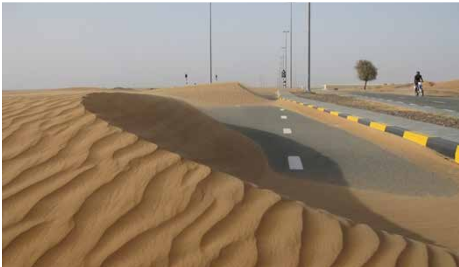
Figure 50. Damage to infrastructure by moving sand dunes
