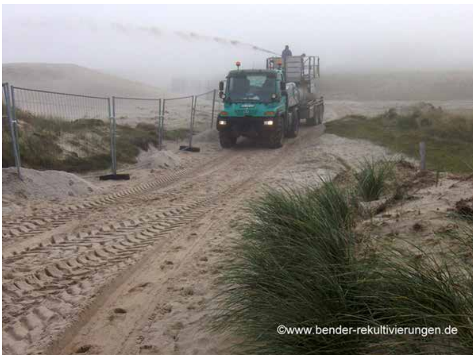
Figure 60. Surface stabilization for dust control at an industrial site using soil binding agents applied by a hydroseeder
